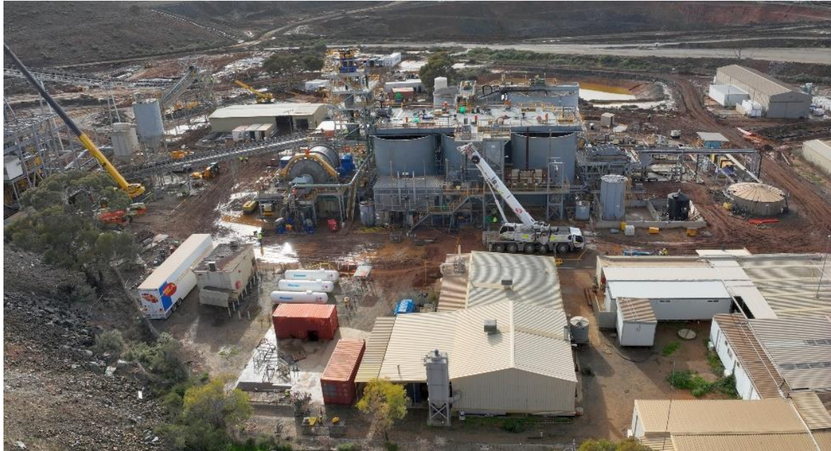
Figure 2: Three Mile Hill Mill refurbishment progress 29 June 2023
