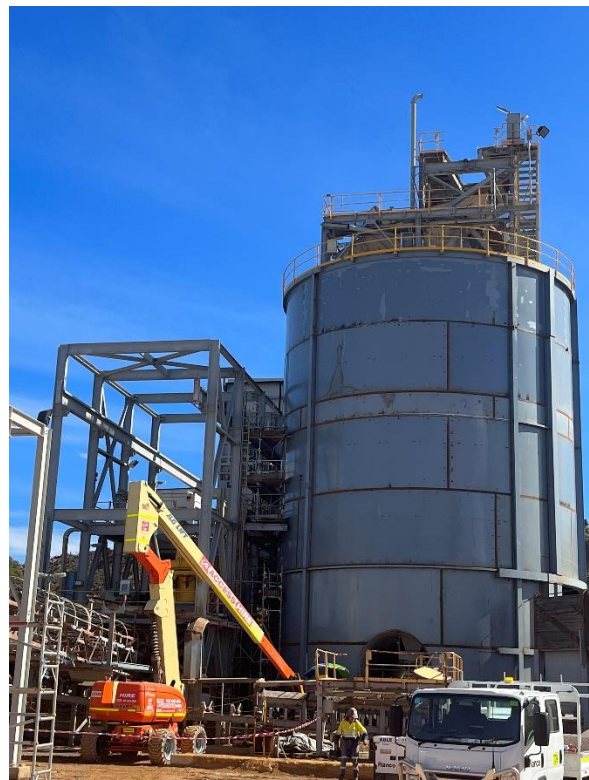
Photo 2: New fine ore bin being erected at site
