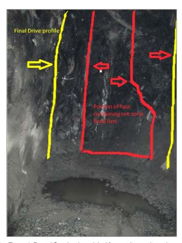
Figure 4: Resue' Cut showing original face and ore only portion of face fired and bogged
