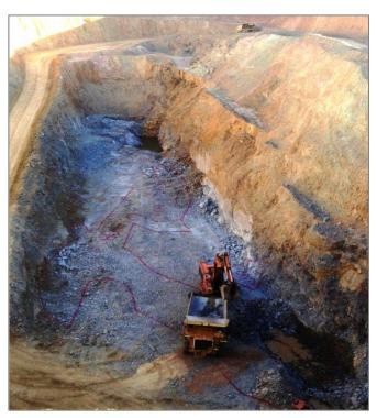
Figure 2: Empress pit showing final floor in far wall under ramp. Ore zones in red paint. Pit has a further 12 metres vertically of ore to be mined from the point shown in the figure.
