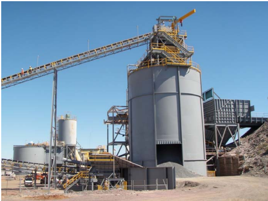
Figure 6: Fine Ore Bin – December 2009
