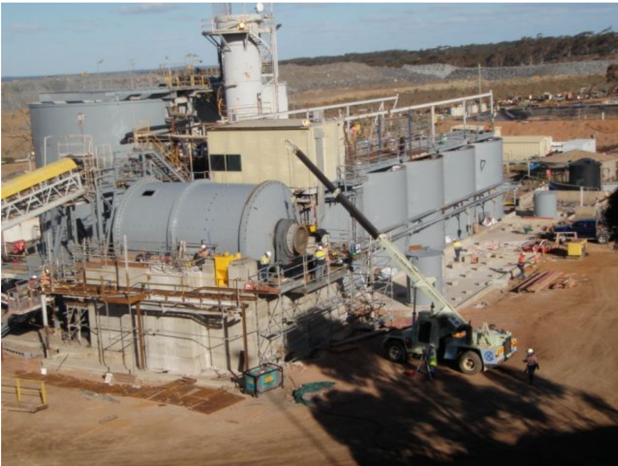
Figure 10: Refurbished Tanks prior to installation of gold room circuits – October 2009
