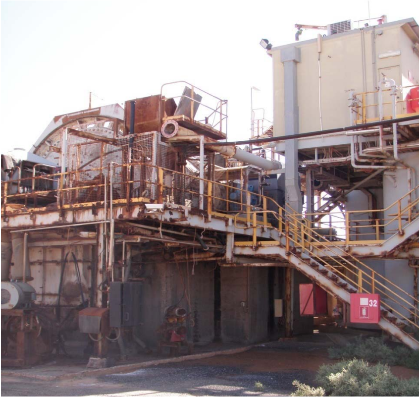
Figure 7: Ball Mill and original foundations – March 2009
