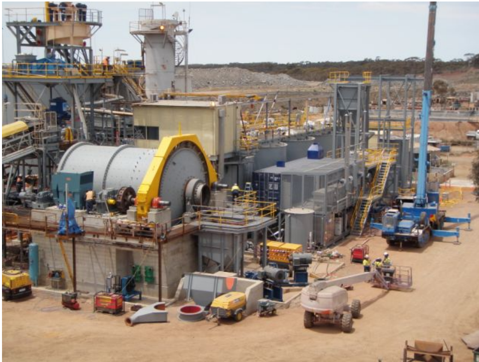
Figure 11: During installation of gold room circuits - October 2009
